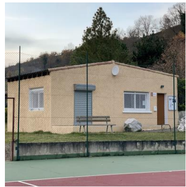
Renovation of the Tennis Club House
